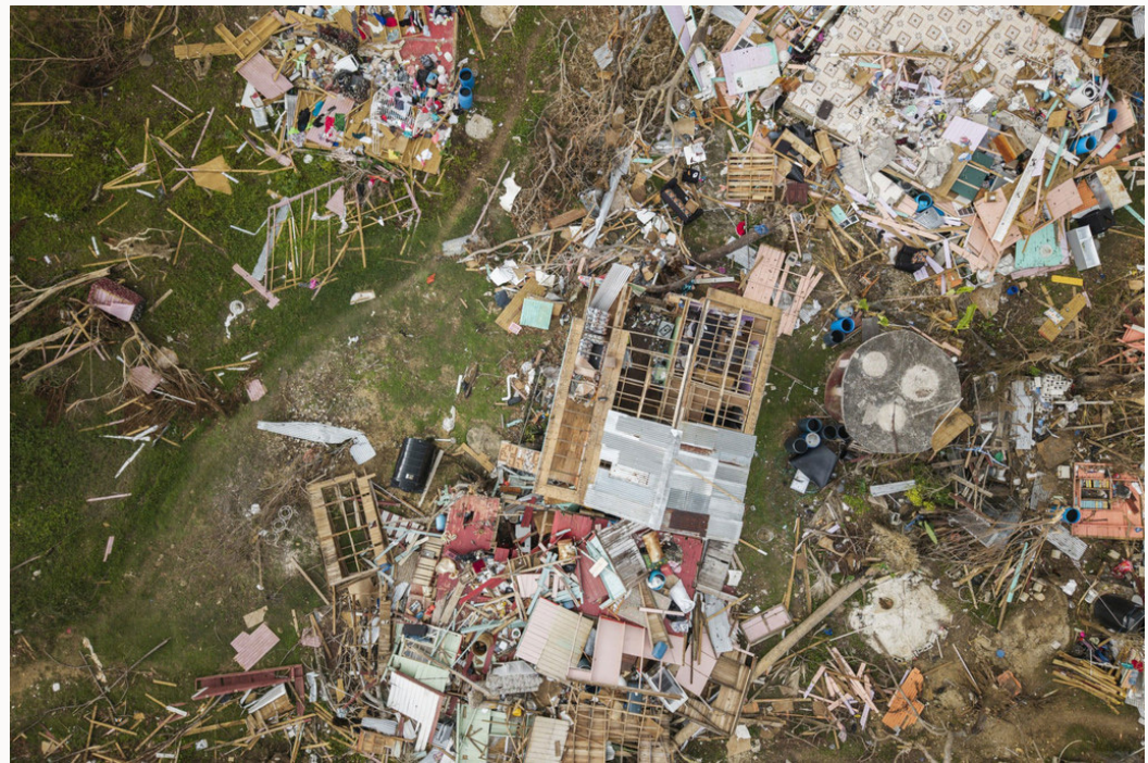
Figure 6. Homes in Westmoreland, Jamaica, were devastated by Hurricane Melissa .
