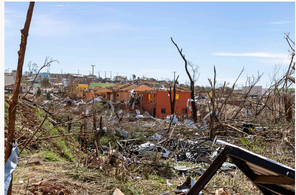
Figure 5. Extensive damage in Rio Bonito do Iguaçu
